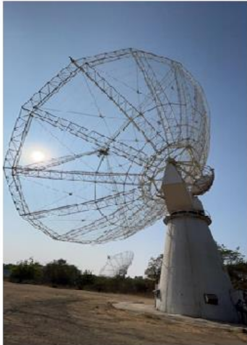
Parabolic dish with an outer diameter of 45m
